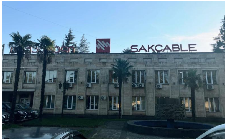
Figure 18: Main entrance of the Sakcable manufacturing facility in Tbilisi, Georgia, where the CPS-II and CCS pilot activities were conducted.
